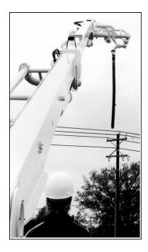
This pumping company used cones and red paint to clearly mark the "danger zone" when electrical wires were within reach of the boom.
