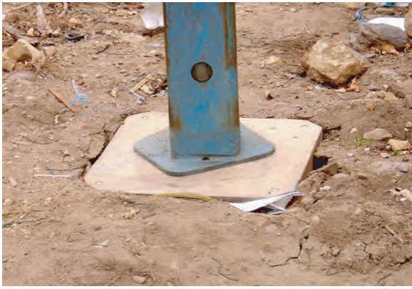
Figure 5 Inadequate cribbing. Is the soil un-compacted or soft?
