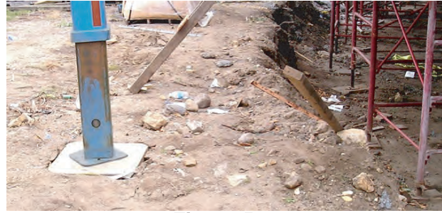
Figure 5 Inadequate cribbing. Is the soil un-compacted or soft?
