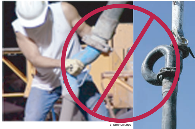
Figure 20 Devices like these weigh too much and pose a hazard
