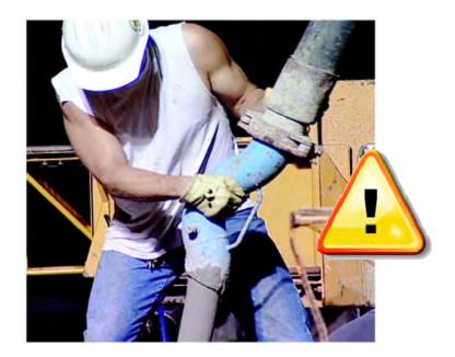
The intended purpose of this device is to prevent concrete from free-falling out of the boom end hose and to create a slower/steadier flow. The use of this device is sometimes requested because it has been shown that concrete loses some of its larger entrained air bubbles upon sudden impact, which could decrease the overall air content.
